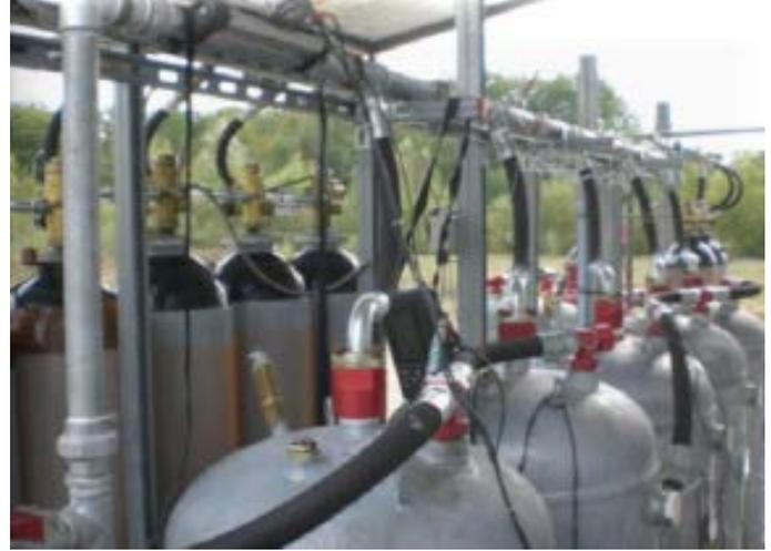
Nitrogen used to deliver water – ©Sinorix H2O Jet - Siemens
