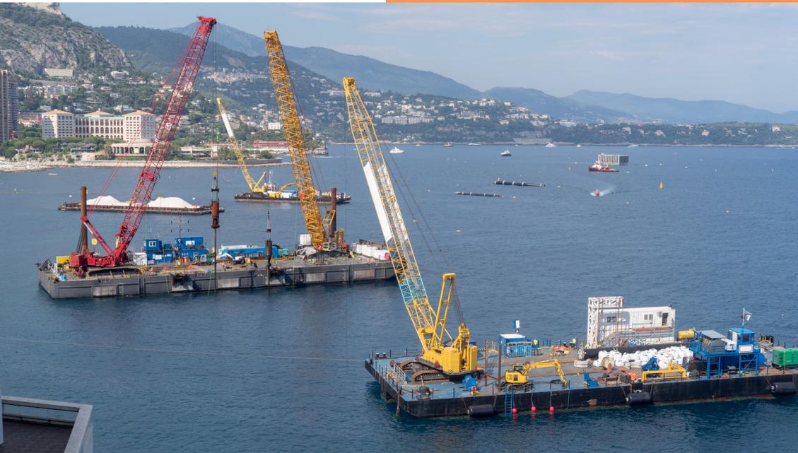
Waterborne exposures for portable cranes and excavators can present additional risks and concerns other than those encountered when this type of contractors' equipment is used on land. Securing the crane so that it does not move while in operation is required. The crane's lifting capacities are generally always reduced, the stability of the barge with a shifting crane load comes into play and the condition and suitability of the barge is a critical factor.
