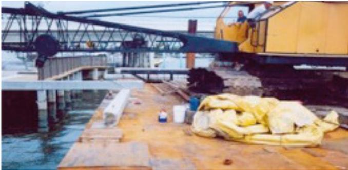
Plywood sheets cover holes in the deck. Also, the crawler crane is not secured.
