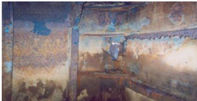
Heavy wastage and deterioration of internal structural members
