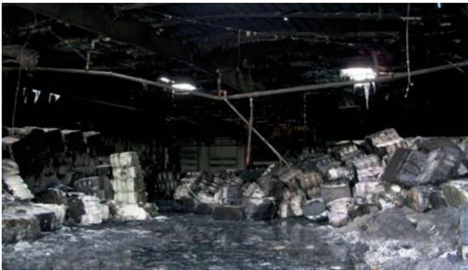
The result of a warehouse with an inadequately designed sprinkler system
