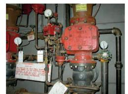
Typical Dry Pipe Sprinkler System and Component Parts
