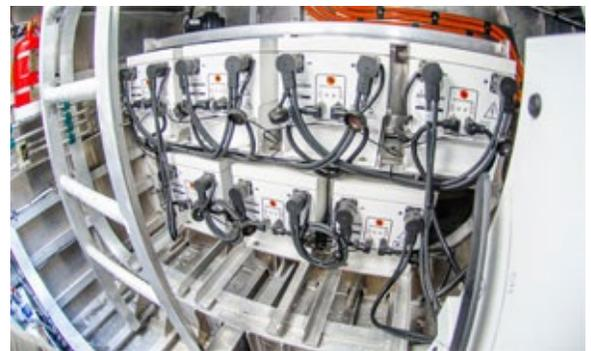
Lithium-ion batteries in a rack on a marine vessel.
