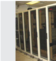
Computer server racks anchored to the floor
