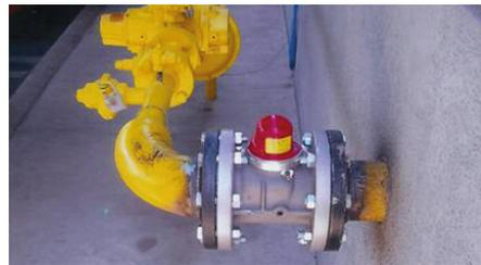
Seismic shutoff valve for natural gas line
