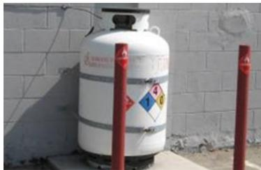
Flammable liquid tank strapped to wall
