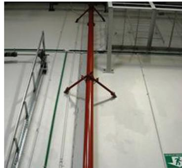
Sprinkler riser with sway bracing
