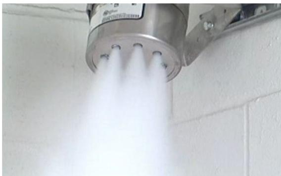
Discharge of a Condensed Aerosol Fire Extinguishing System.
